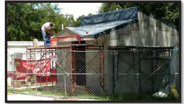
New ADA-compliant restrooms at Lake Alfred Elementary.
