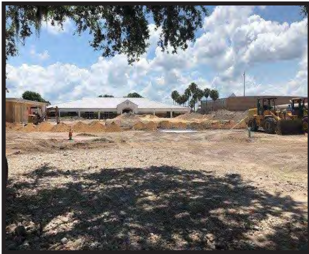
Bartow High School Renovation.
